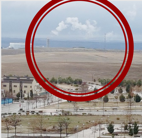
Valdemingómez waste incinerator
